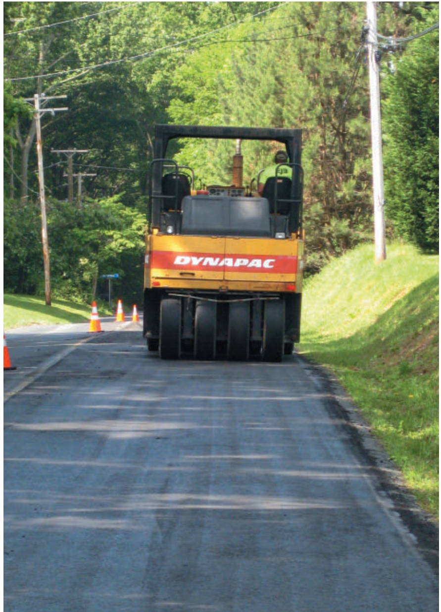
In Limerick Township, 22-30 ton pneumatic rubber tired roller provides compaction
