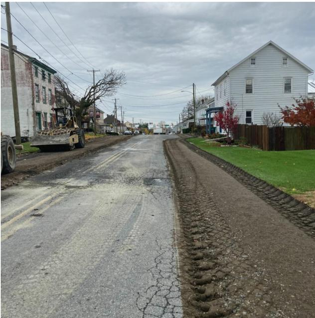
types of roads often do not get the adequate base needed to support the road structure. For this neighborhood, Bethel Township reinvested in the existing pavement & subbase through Full Depth Reclamation (FDR) with cement.
